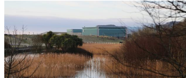
Arklow Wastewater Treatment Plant upgrade - €139m (complete)
