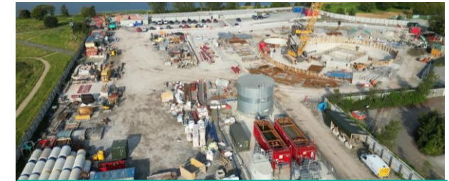
Athlone Main Drainage Scheme - €114m (wastewater, complete)
