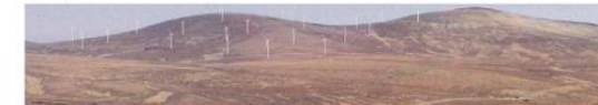
1(b) Wind energy development with many turbines of medium height - this can be inappropriate. The spatial extent of a wind energy development can be reduced by using taller turbines. This may be a preferable solution in some situations.
