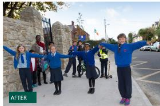
New widened footpath (Photo: DURCC)
