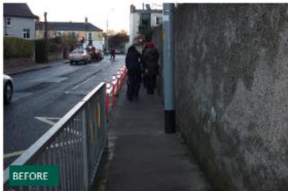
Narrow footpath on Convent Road (Photo: DURCC)
