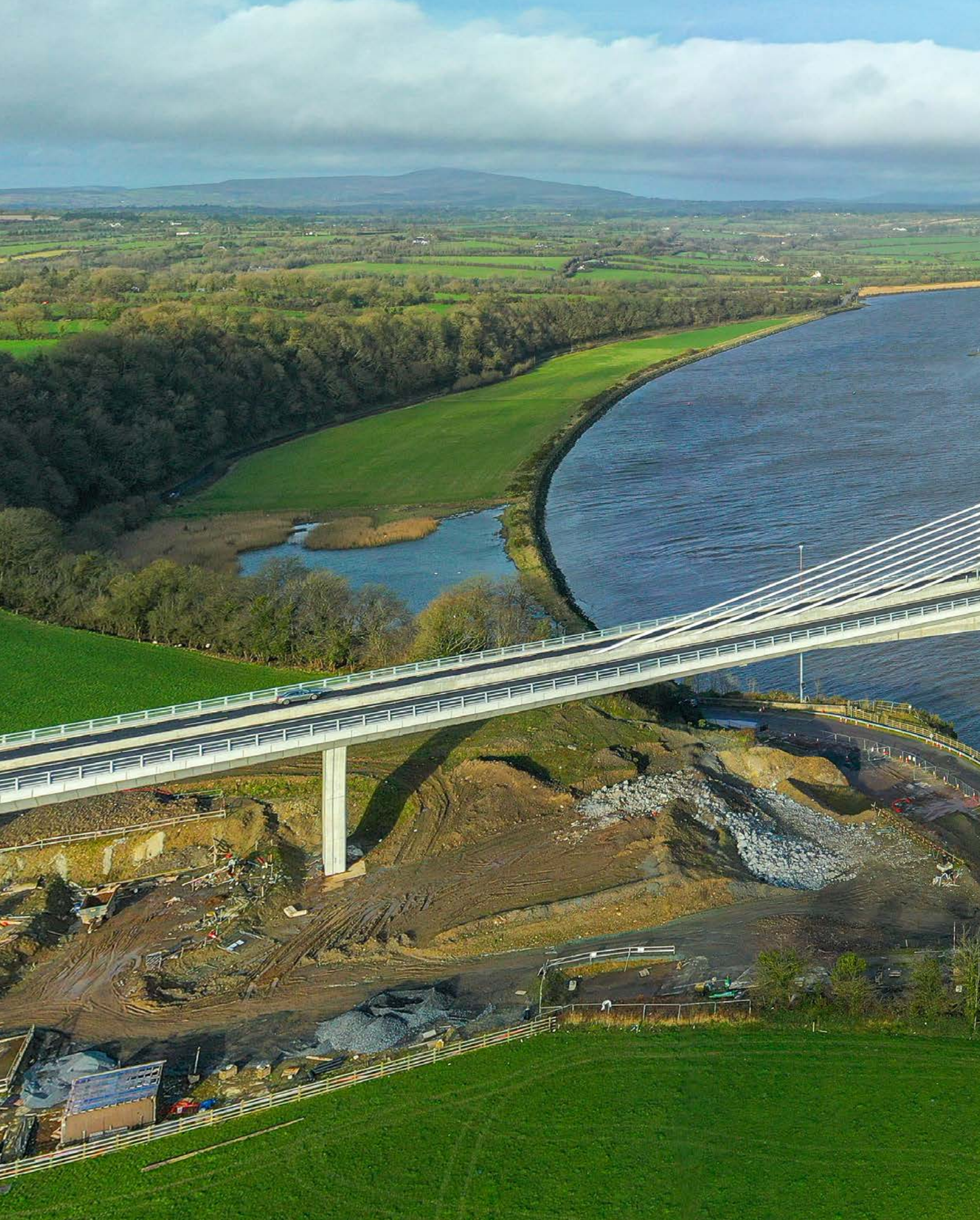
Rose Fitzgerald Kennedy Bridge, Co Wexford
