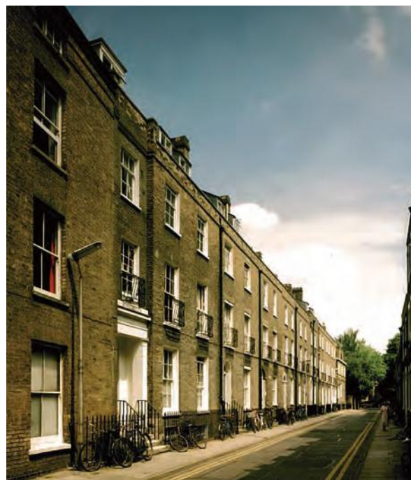
Figure 3: In Georgian streets the small spacing-to-height ratio is compensated for by tall windows. Note how window head height increases for the lower floors which are more heavily obstructed.
