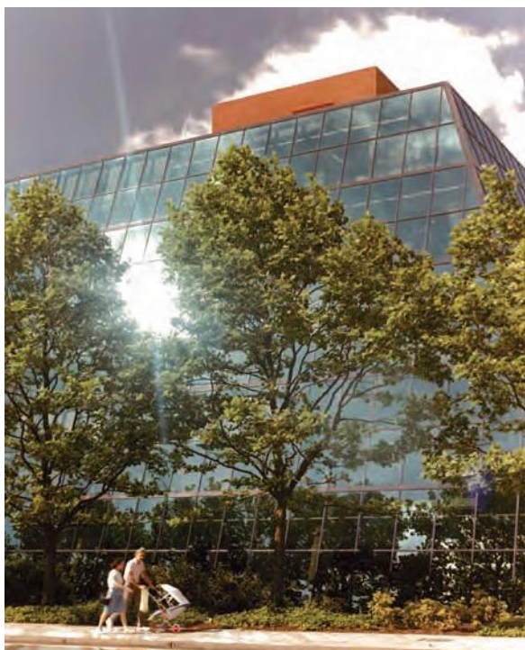
Figure 39: Solar dazzle reflected from a glazed façade
