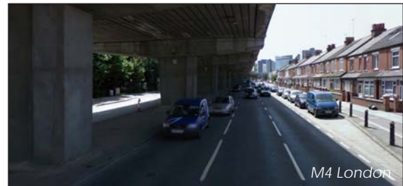
Figure 3.30: Examples of major urban roads that move large volumes of traffic via vertical segregation. These require significant investment in infrastructure. As illustrated in the middle and bottom examples they can have negative impacts in terms of place and/or connectivity (image sources: Google Street View).
