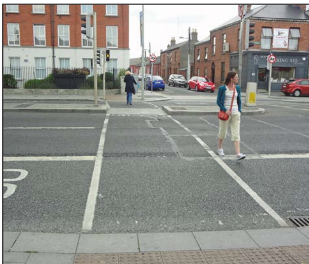
Figure 4.39: Example of a wide streets with a crossing that allows pedestrians to cross in a direct manner and in a single movement. The median acts as a refuge island for those users who cannot cross the street in a reasonable time.
