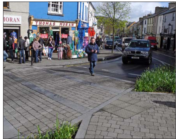
Figure 4.38: Example of an informal 'courtesy' crossing in Westport, Co. Mayo. Drivers stop and wait for pedestrians to cross as a courtesy.
