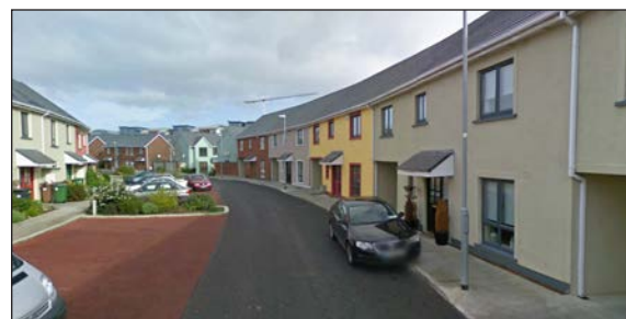
Figure 4.65: Example from Clongriffin, Co. Dublin where a change in the alignment of the street calms traffic as drivers proceed cautiously due to the uncertainty of what lay ahead (image source: Google Street View).
