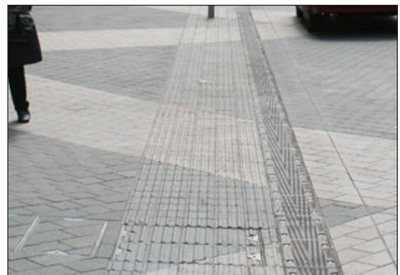
Figure 4.74: Example of an drainage channel on Exhibition Road, London. The kerb line indicates an area of pedestrian refuge and is used to guide the visually impaired.
