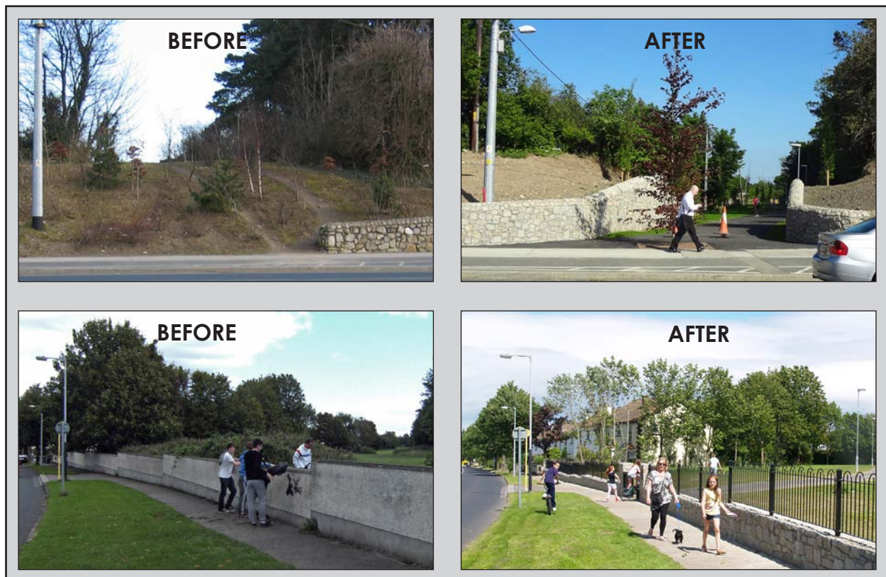
Figure 3.12: An example of two local permeability projects in Dublin which have significantly improved local access to the LUAS (top) and local shops (bottom) for pedestrians and cyclists. These links formalised routes that were used by locals which previously involved walking across unlit fields, muddy patches and/or climbing over/through fences.
