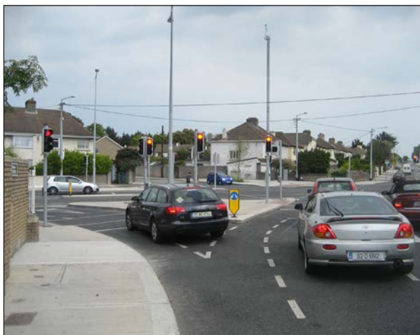
Figure 4.59: Left turning slips (left) generally offer little benefit in terms of junction capacity and increase the number of crossings pedestrians must navigate. They also allow vehicles to take corners at higher speeds, exposing pedestrians and cyclists to greater danger. Where a large number of turning movements occur, left turning lanes (right) with tighter corner radii should be used.
