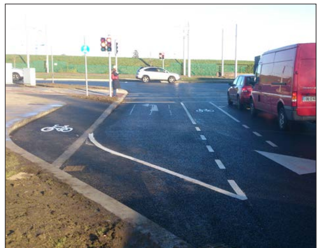
Figure 4.59: Left turning slips (left) generally offer little benefit in terms of junction capacity and increase the number of crossings pedestrians must navigate. They also allow vehicles to take corners at higher speeds, exposing pedestrians and cyclists to greater danger. Where a large number of turning movements occur, left turning lanes (right) with tighter corner radii should be used.
