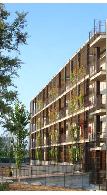
The key is to have offset gallery access from the units as shown in the project with mini bridges reaching over to the doorways of each unit. Typically kitchens and bedrooms are located on the gallery facade.
