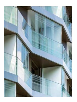
Image showing glazed floor to ceiling panels in balconies.
